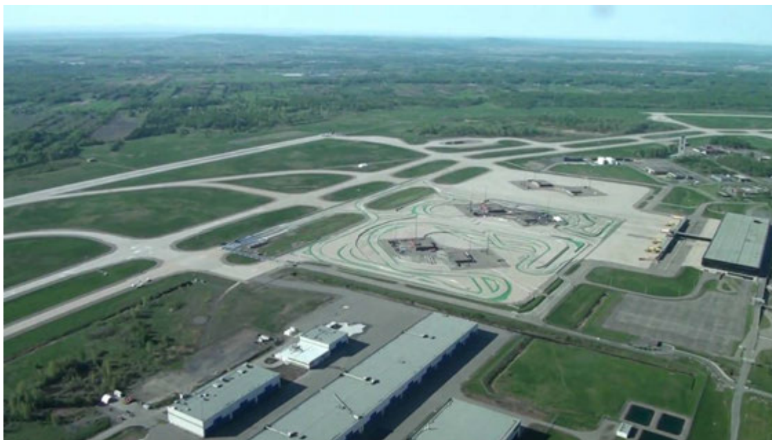
Montreal Mirabel International Airport Built for the 1976 Olympics
