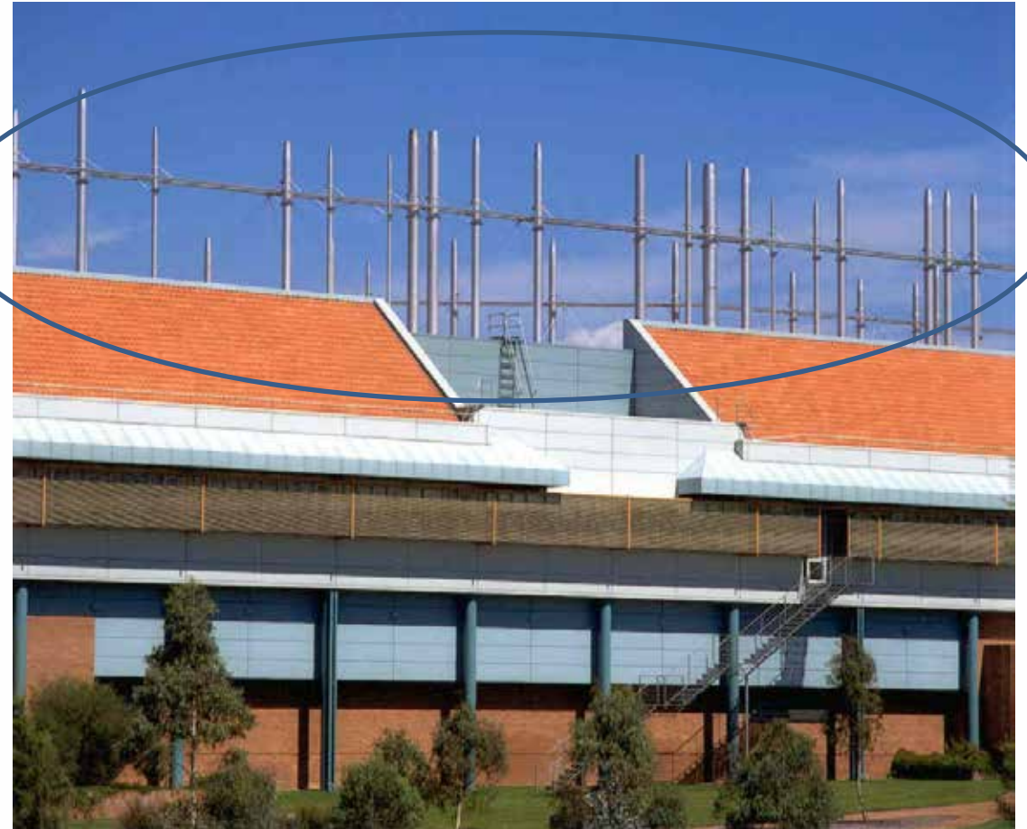
Purpose built science and engineering building
