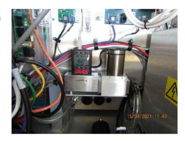
The flow meter was photographed prior to extraction so that it could be re-connected upon return. Before shipment it wrapped in plastic to safeguard against contamination and wrapped in bubble-wrap before placing in a box with sufficient cushioning to prevent damage by couriers during transport.
